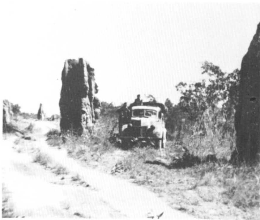
On the Southport Road: Various attempts were made to upgrade the Southport Road, but the wet always won.
